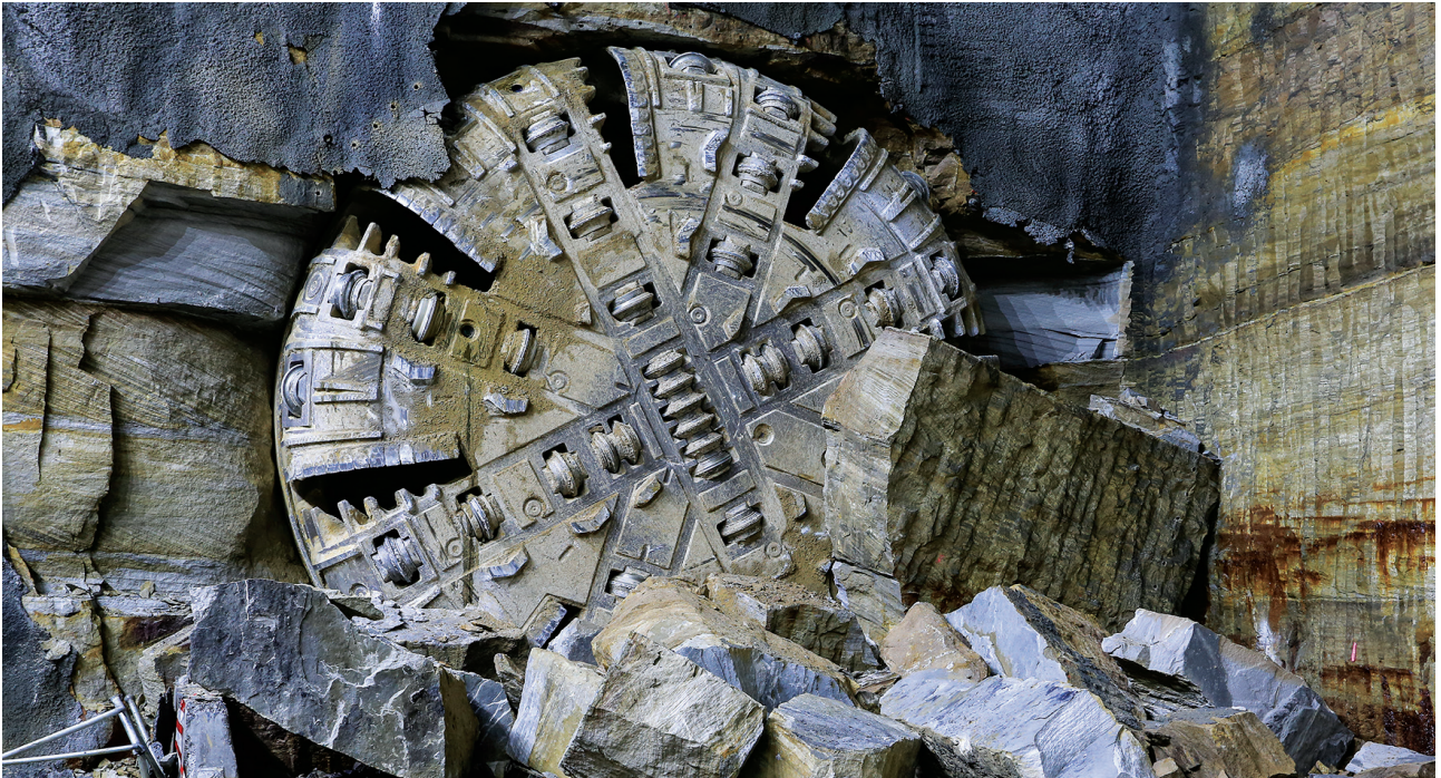
Break-through: Tunnel Boring Machine 2 Florence arrives at the Showground station site. Photo courtesy of Transport for NSW.
